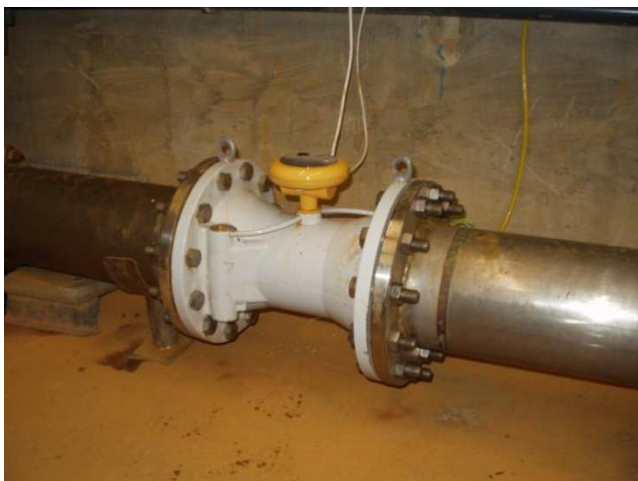
Installation of the battery-powered ultrasonic water meter FLOMIC FL 1024 in a station
