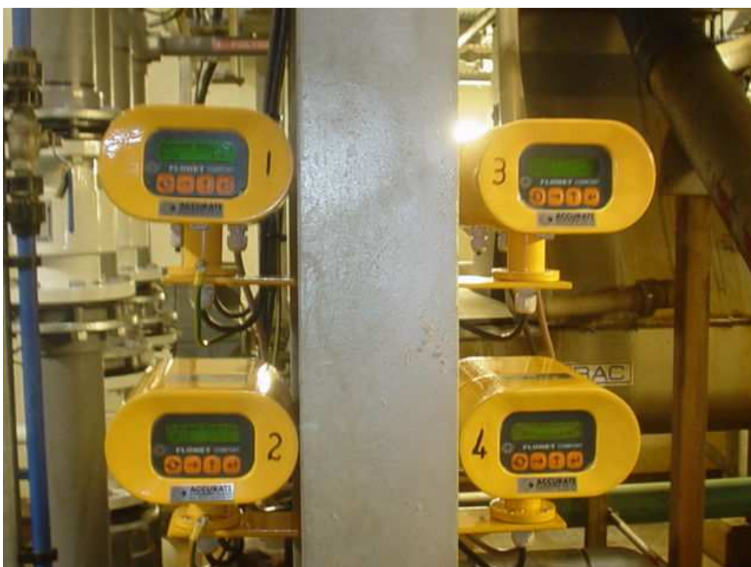
Electronics of induction flow meters FLONET FN 2015 in remote version
