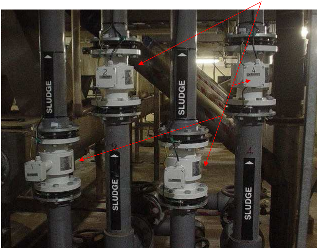
Sensors of induction flow meters FLONET FN 2015.1 in remote version DN 125/PN 16
