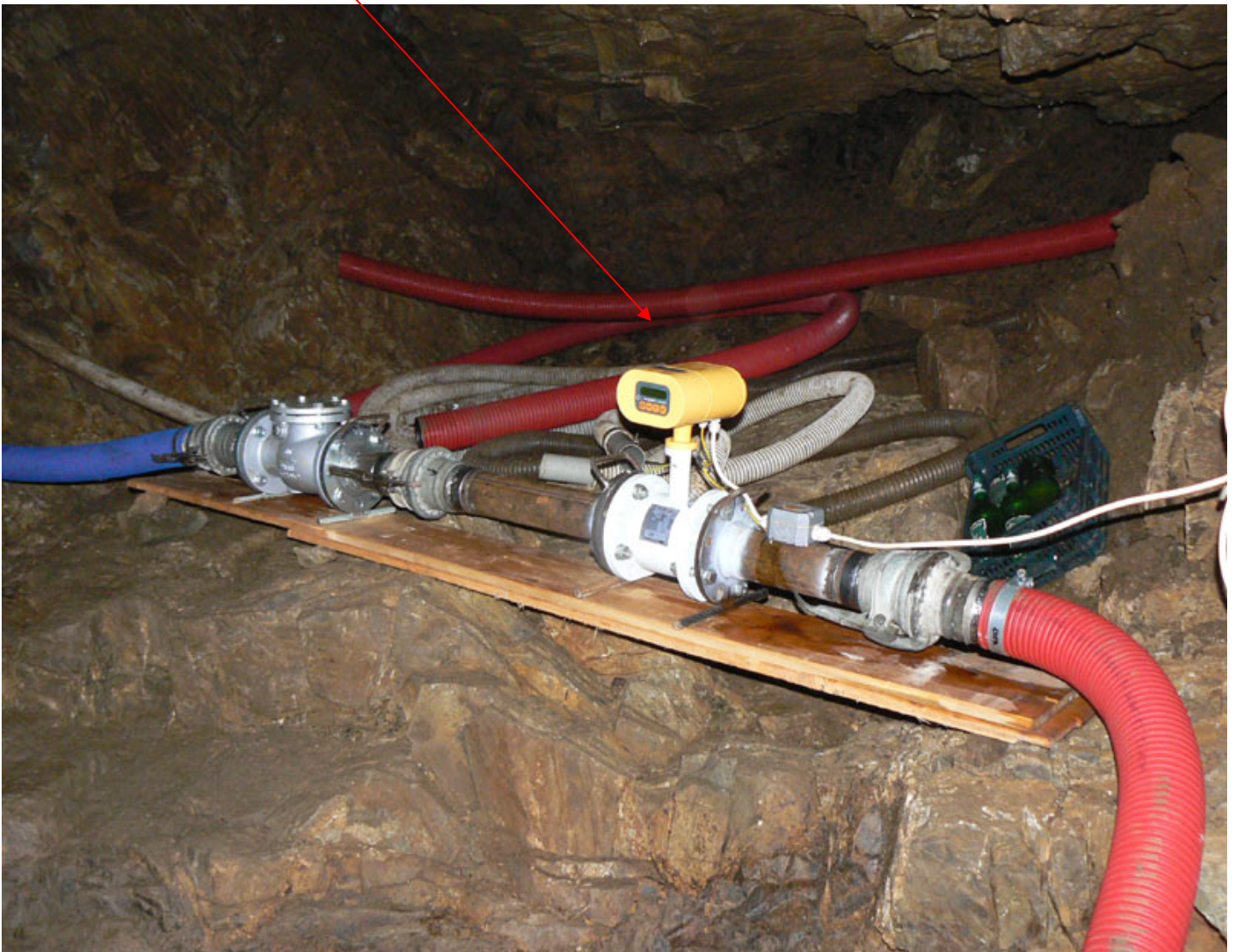
Induction flow meter FLONET FN2014.1 DN 80/PN16
